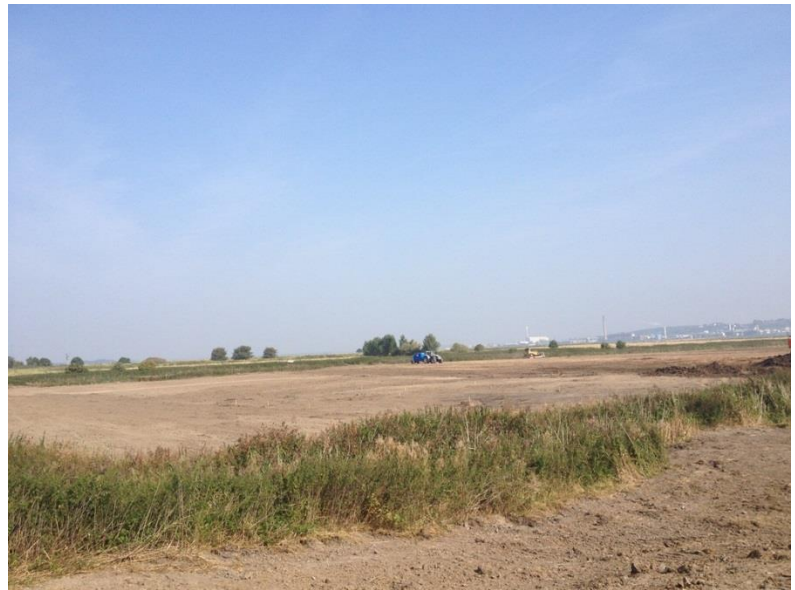
Photo: Cell 3 following clearance and levelling
