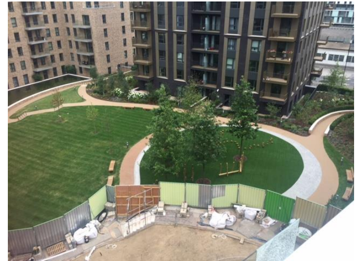
The podium garden showing completed sections and areas still under construction.
