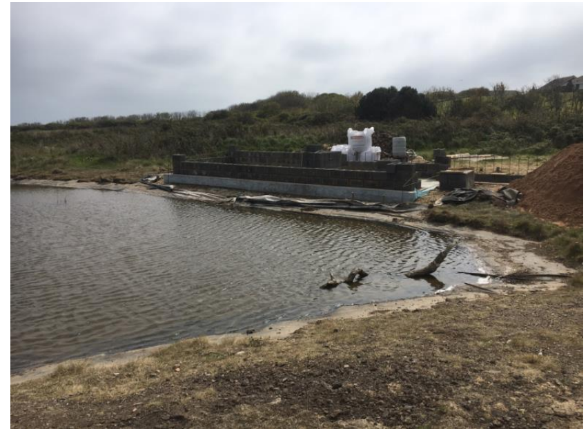
Ongoing construction of the nesting bank
