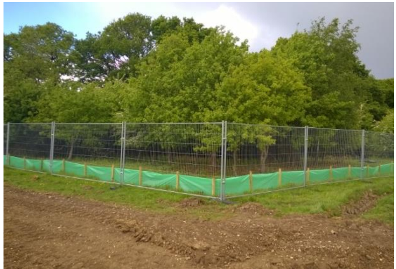
Photo: Area TPO protection and reptile fencing
