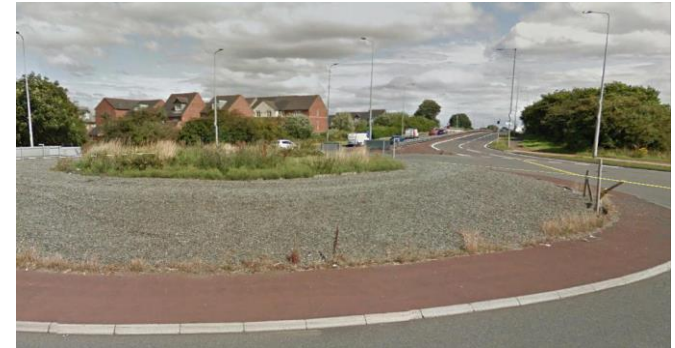
The Golborne East Lancs Roundabout before:
