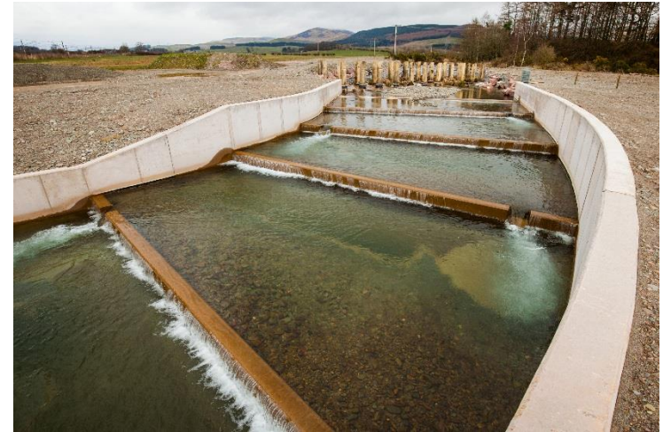
New channel base levels
