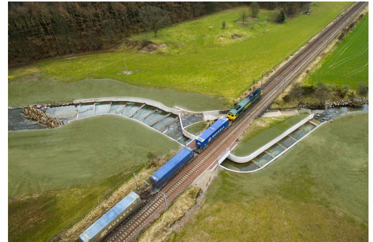
Aerial photograph of the new fish pass
