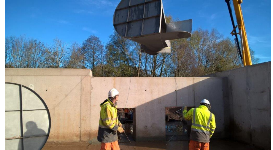
Hydrobreaks being added to new flood channel
