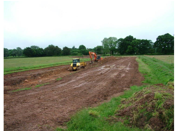
Groundworks start for new flood channel
