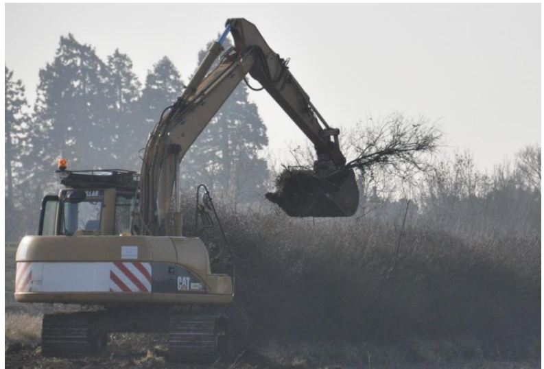
Photo: Lifting existing hedgerow for use in reinstated hedge
