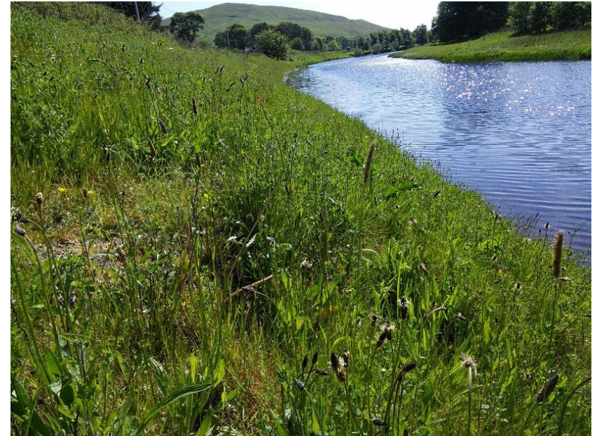
Photo Description: Lamington Viaduct Embankment – May 2017.
