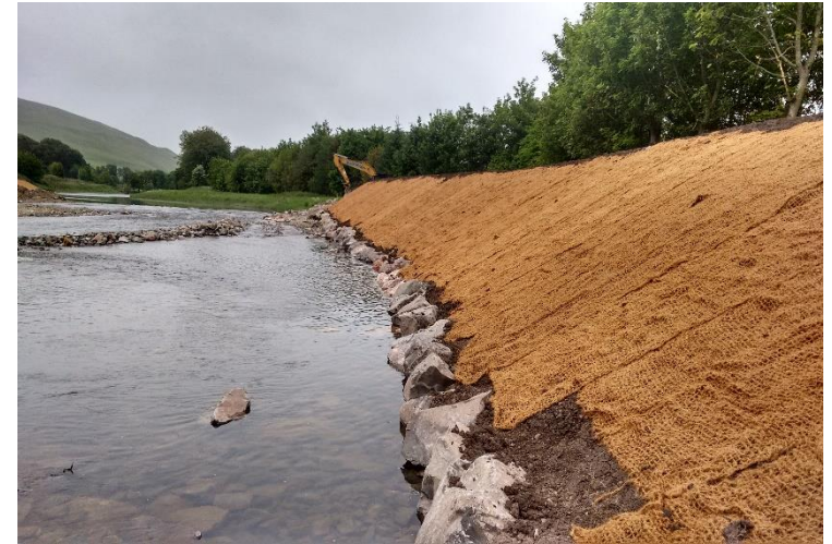
Photo Description: Construction of the embankment - July 2016
