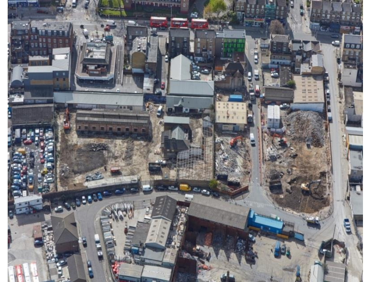
Aerial photo of site taken during demolition works
