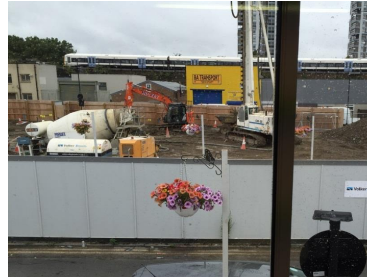
Pensbury Street showing Hard Hat hanging baskets in place.
