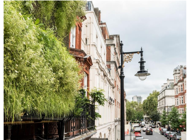
Living wall in full growth Credit: Arup
