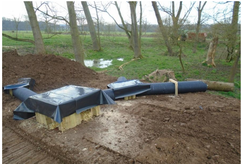
Photo: New Badger Sett Underconstruction
