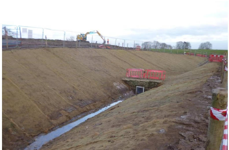
Photo: Completion of installation of pre-seeded matting
