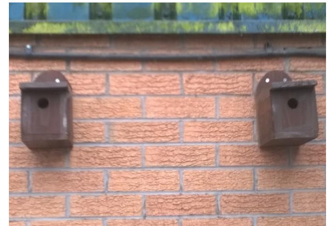
Two of the 6 bird boxes fixed to an exterior wall in our Falkirk Depot.
