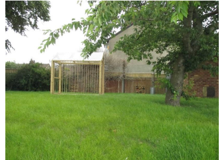
The Environmental greenhouse under construction.
