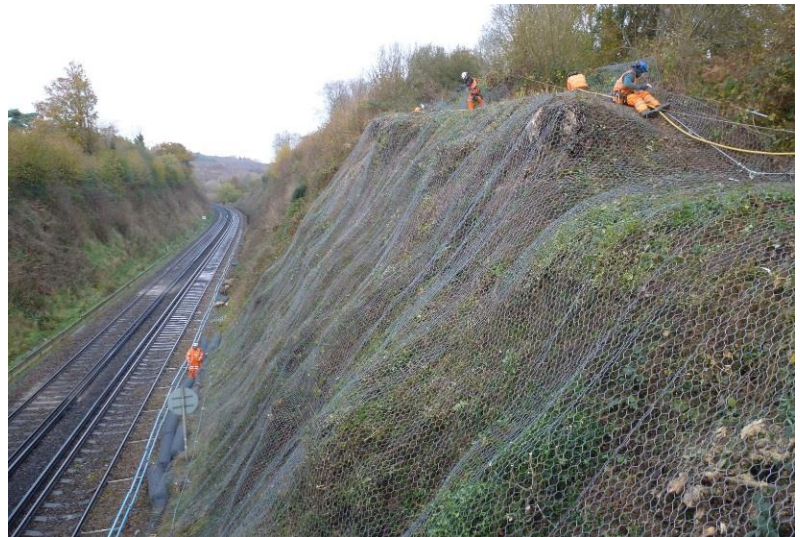
Photo: Embankment stabilisation at Scrag Oak
