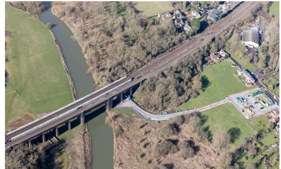
Ariel view of the viaduct and compound
