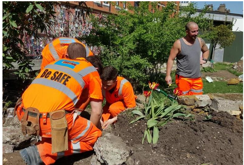
Photo: Costain volunteers at brick laying workshop
