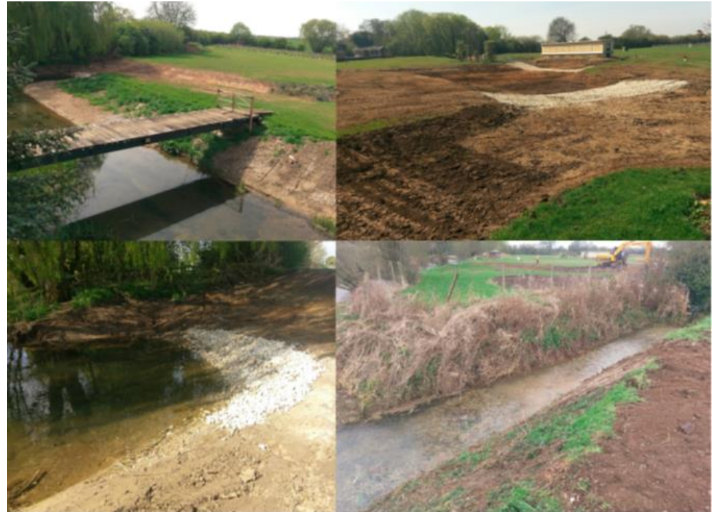
Photo Description: Left top/bottom – New River Embayment and pool. Top Right – New swales in the main field area in front of the sand martin house. Bottom Right – New Riffle followed by a pool on the ditch river outfall.
