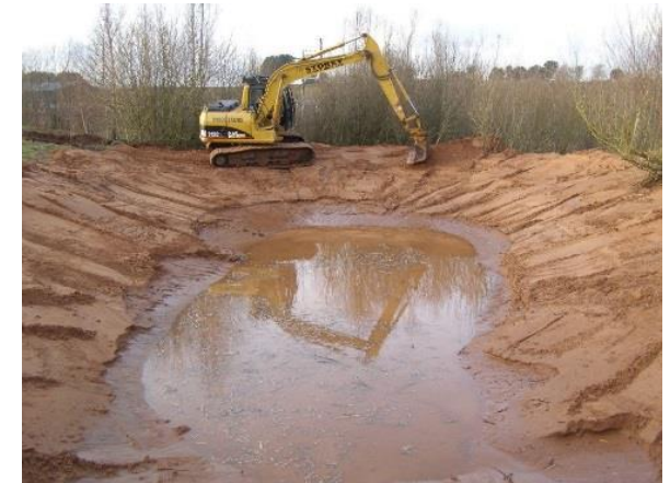
Pond creation at Crown Farm Quarry
