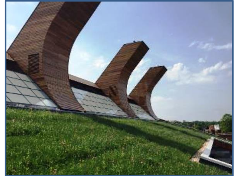
Photo Description: the completed wildflower roof.
