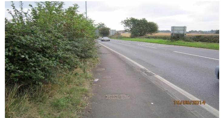
An image of the narrow footpath and adjacent hedgerow prior to the start of works
