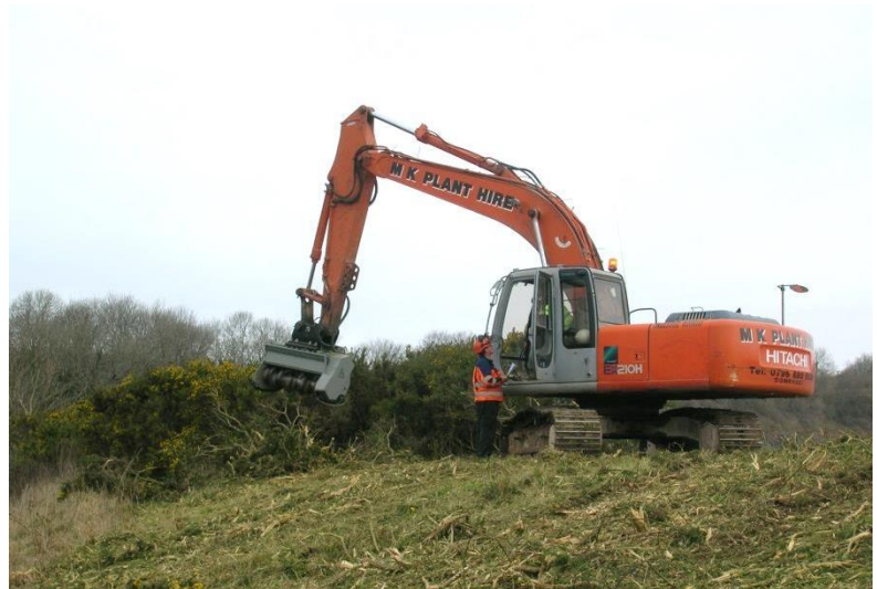
Photo: Scrub clearance
