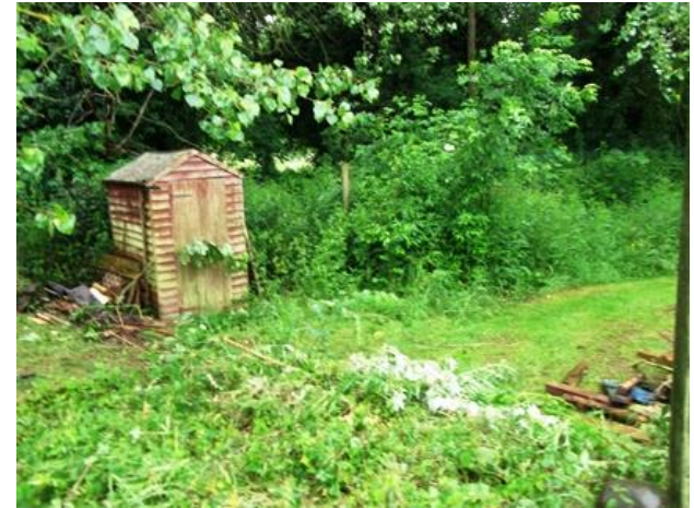
Old fence gone. Shed to follow.
