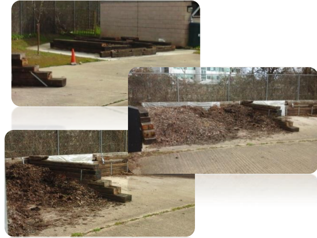
Construction of raised sleeper beds
