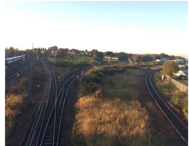
The Triangle prior to any works
