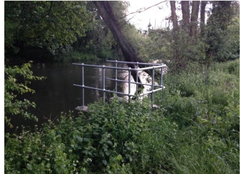
The headwall intake and sluice gate off the River Kennet after construction. A buried pipeline connects into a ditch at the head of the reedbeds.
