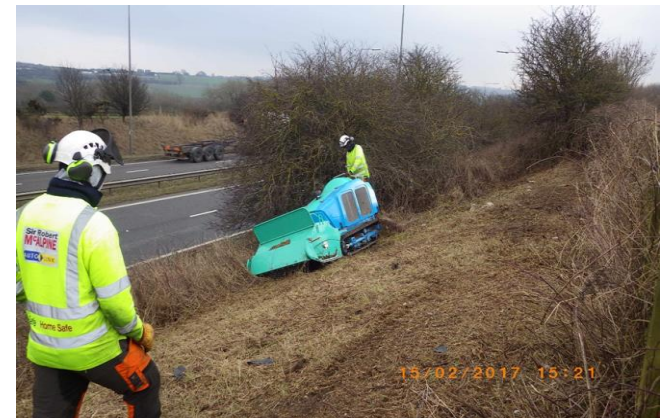
Highway embankment scrub clearance (Sir Robert McAlpine)
