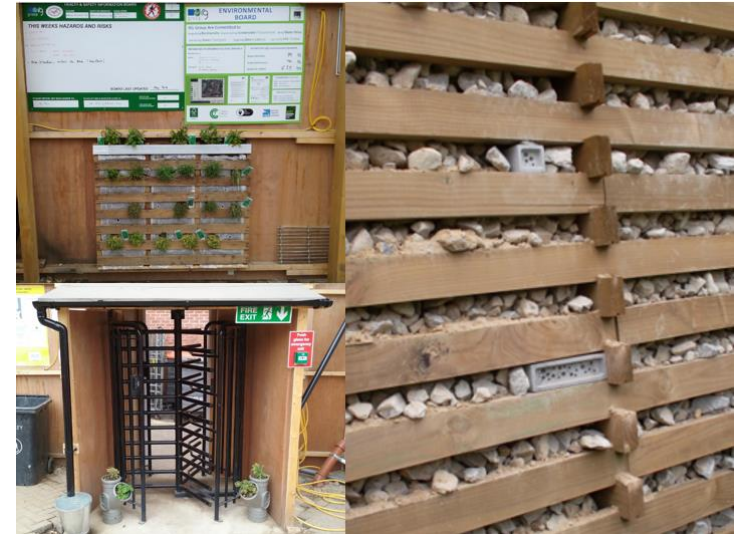
Top: site environmental board with herb garden underneath; bottom: turnstile entrance with planted pipes which were off cuts; Right: retaining wall with bee bricks in situ
