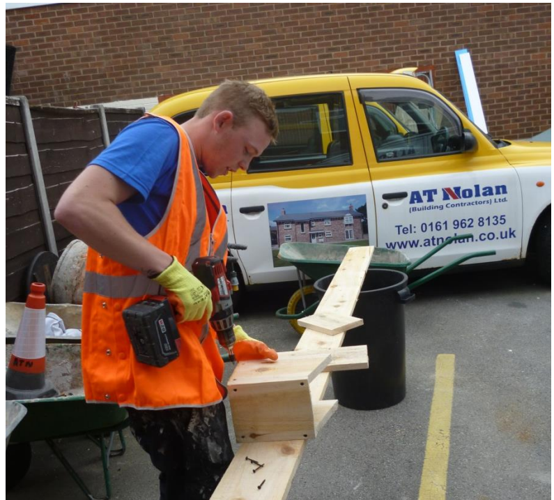
Photo: Box construction
