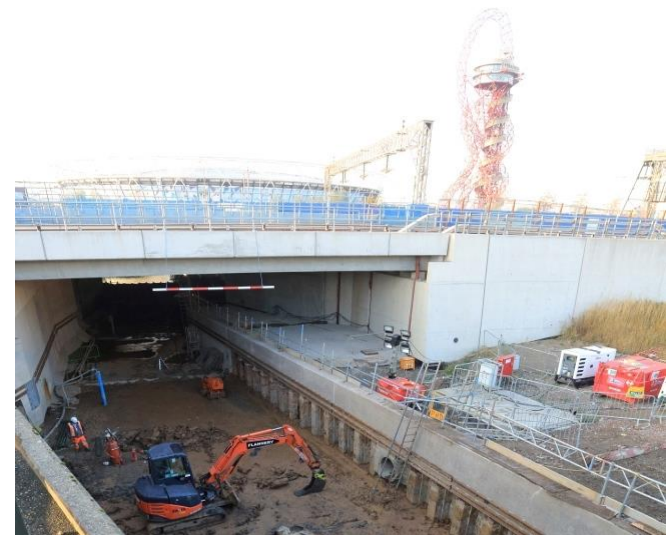
City Mill River Works – Backdrop of Olympic Park
