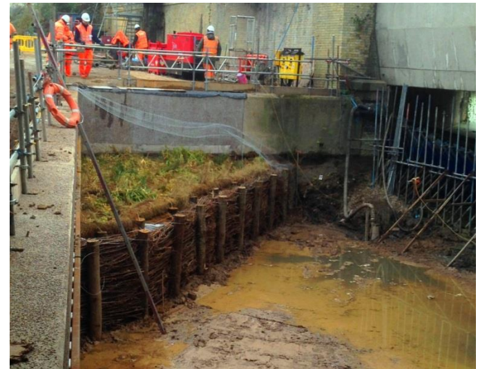
Installation of reed bed while river dammed & being dewatered
