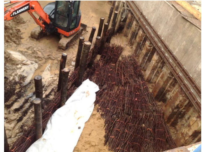
Brushwood being installed within Chestnut stakes
