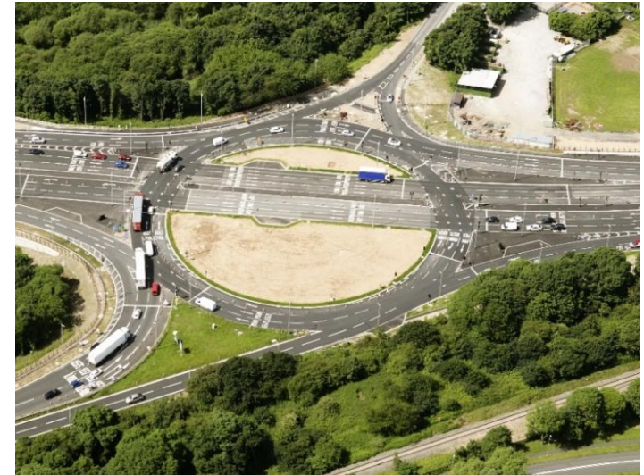
Receptor site: M56 J12 Roundabout (BEFORE)
