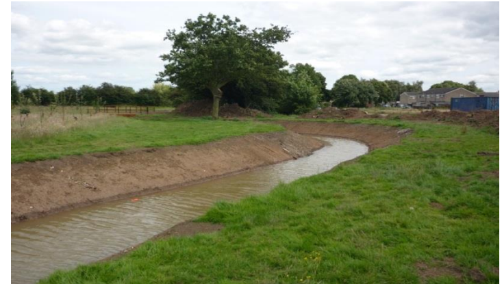
Daylighting of the culvert with a meandering bend around the existing trees
