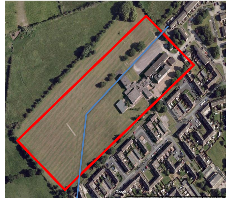
Existing site before demolition of the school, blue line indicates existing culvert
