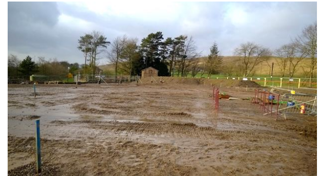
Site clearance for groundworks preparation (Sir Robert McAlpine)
