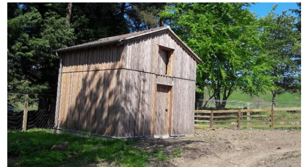
Pre-demolition dual-purpose ‘bat hotel’ and cycle storage (Sir Robert McAlpine)
