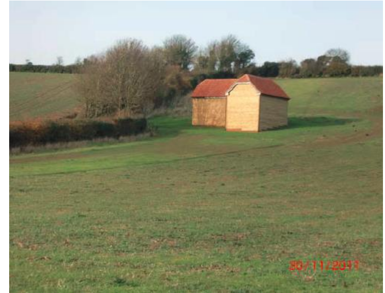
Purpose built bat barn
