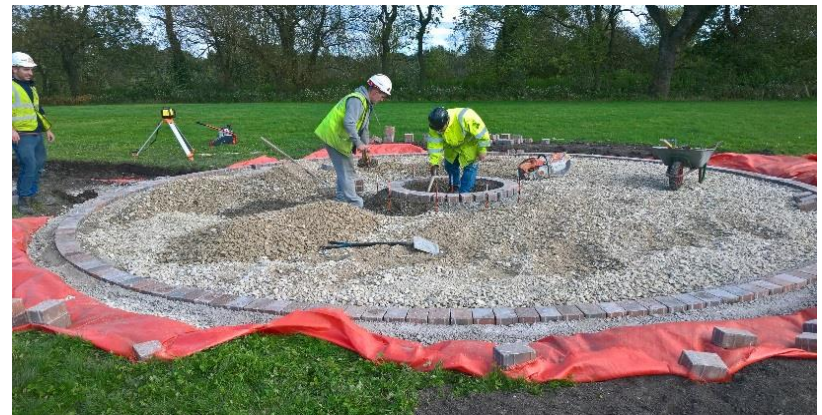
Path / seating area installation
