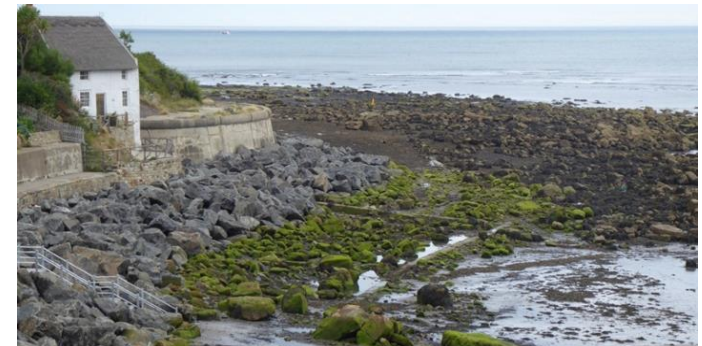
Runswick Bay CDS. The green boulders are the existing boulders which were used to "seed" the new defence
