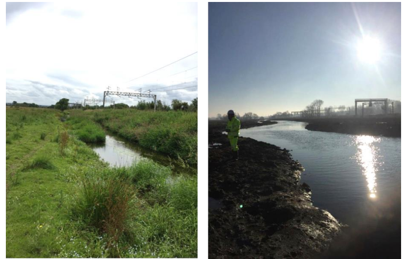
Before & After Image of River Sow Re-alignment Works
