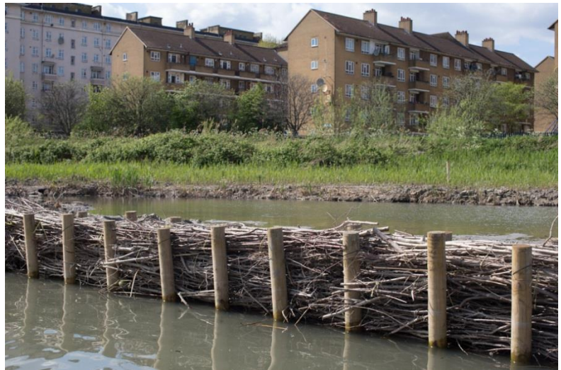
Photo: Chestnut and Hazel revetments in place
