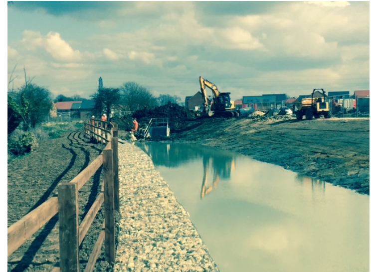
Work gets underway to create Linear Park
