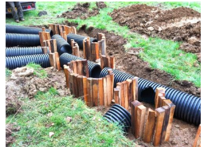
Artificial badger sett constructed as compensation to replace a sett that had been closed
