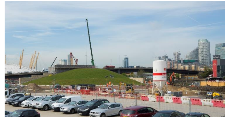
Completed green mound.
