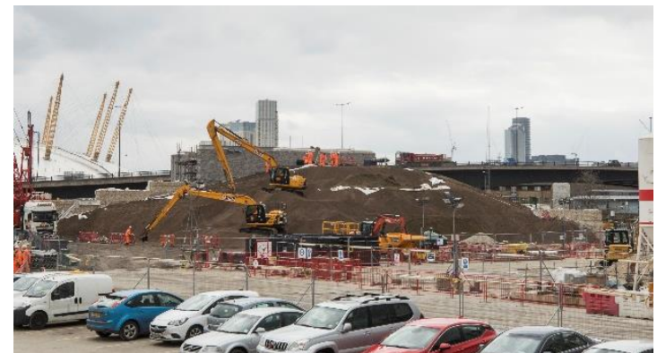
Positioning lytag into mound shape.
