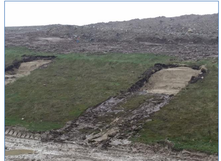
New homes for the sand martins - vertical sanded faces cut into an existing embankment, providing an ideal home for a nesting sand martin
