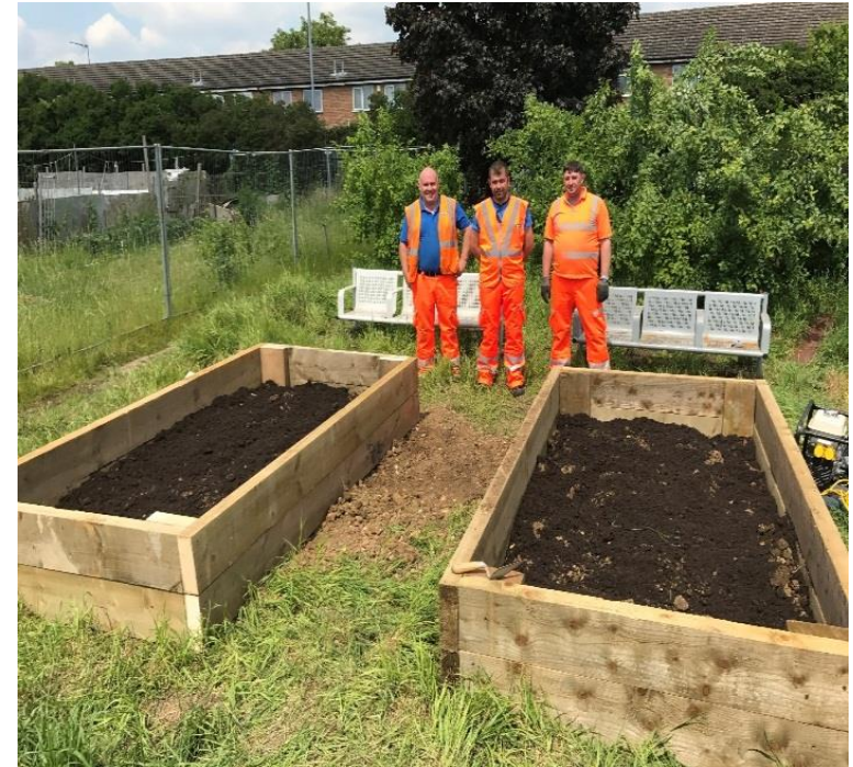
Murphy staff working on the planters
