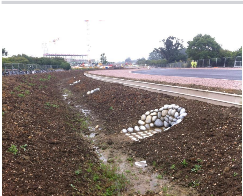
Photo: Newt fencing with swale construction
