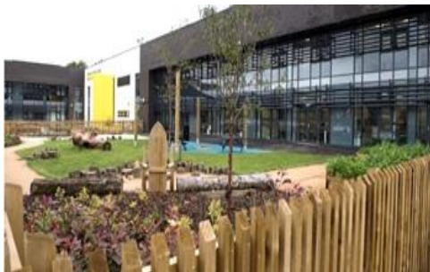
Whittriggs Primary School, Morrison Construction & Ayrshire Council
