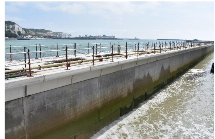
Figure 4. DWDR: New Habitation on Textured Concrete Surface at Marina Pier
