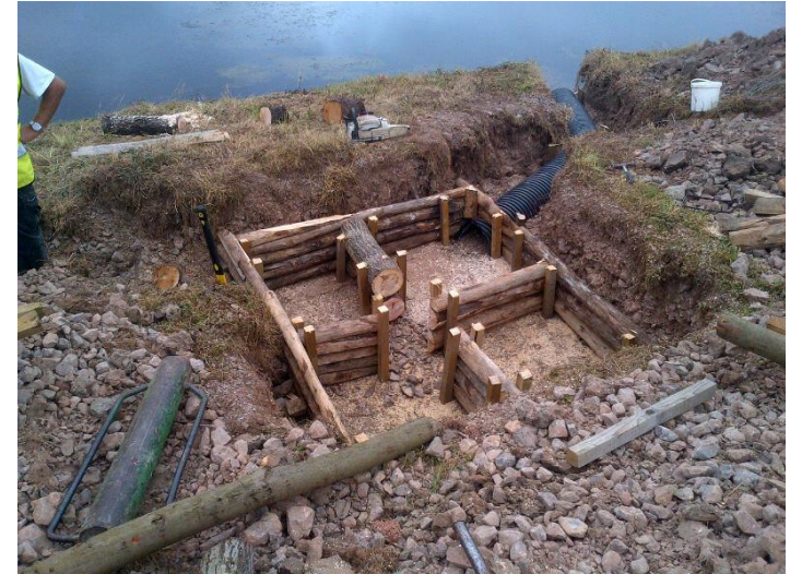
Artificial otter holt part-way through construction
