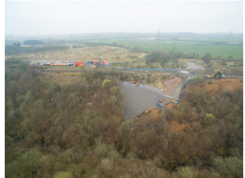
Works progressing on site, with approx. 75% of the new embankment complete:
