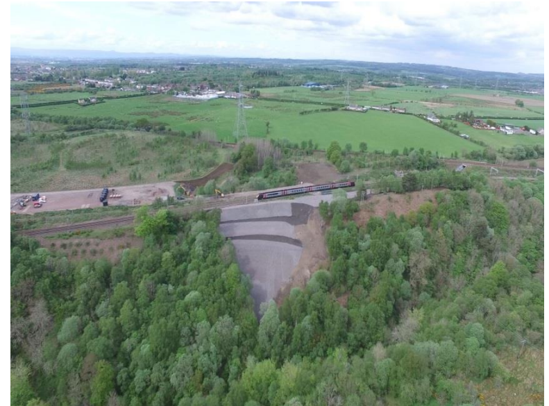
Completed works showing new embankment profile:
