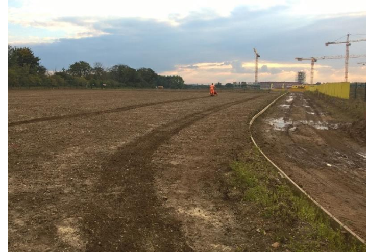
Ground preparation works
